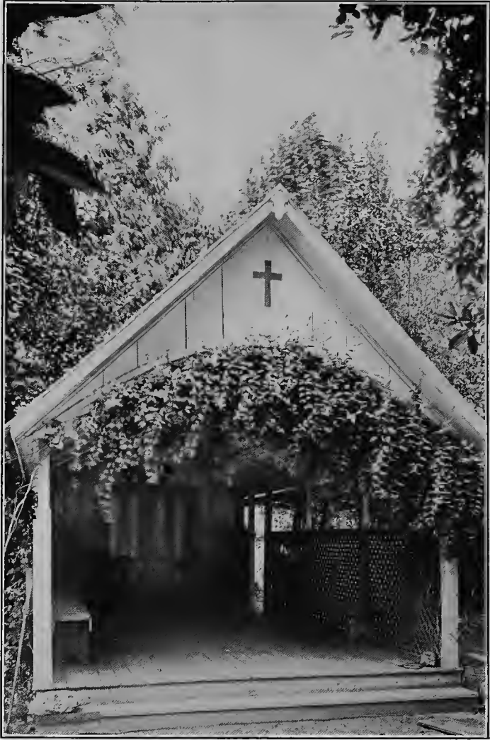
ARCADE ENTRANCE TO CHAPEL, CAMULOS
